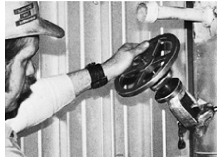
After tool locknut has been tightened against yoke face, to prevent too deep a bite into seat material, seat can be reconditioned by means of a series of five or six slow cuts.
